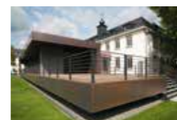
BMAS, Canteen Building V, Bonn pbr, Planungsbüro Rohling AG, Osnabrueck KME Architectural Solutions, Osnabrueck TECU® Classic_bond
