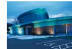
Centrum pomocy chorym na raka Maggie's Highlands Cancer Caring Centre at Raigmore Hospital, Inverness, GB Page & Park Architects, Glasgow W B Watson Ltd., Stewarton TECU® Patina, TECU® Oxid
