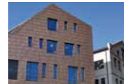
Granary Wharf – Abbey Road, Barking, UK Pollard Thomas Edwards Architects (PTE), Londyn, UK Roles Broderick Roofing Ltd, Chobham, UK TECU® Bronze
