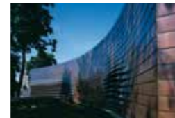
Centrum kultury, Chateau-Rouge, Annemasse, F Cabinet R. Plottier, Lyon Ets. Fourquet, Perouges TECU® Classic
